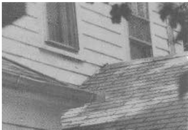
Figure 4. Here, siding that was perfectly good for 30 years is deteriorating from being cut into during renovations and left unsealed.
