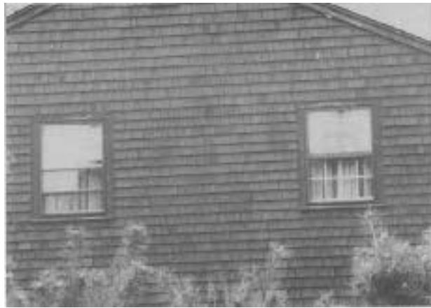
Figure 7. Despite being stained three times, these five-year-old white-cedar shingles are badly curled, and water is reaching the sheathing. Shortly after, the house was vinyl-sided.
