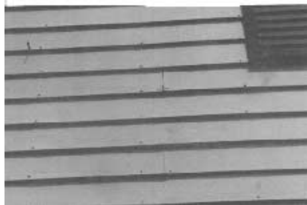
Figure 8. If unprotected, the bottom (butt) edge of hardboard siding will absorb rain and dew up several inches (center photo). Once wet, the material will expand over the nail heads (bottom photo) and sometimes delaminate.
