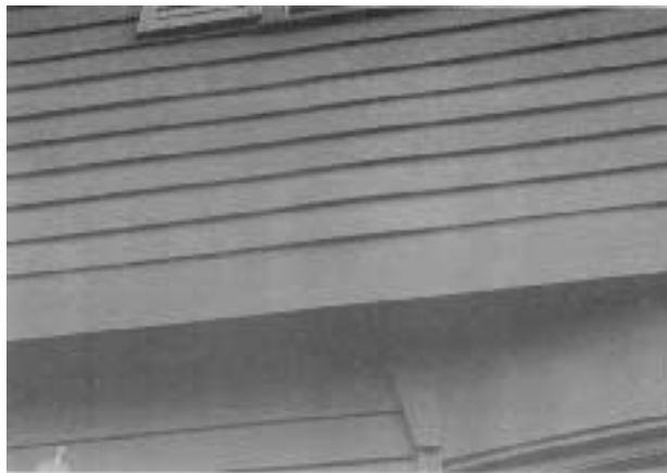
Figure 9. Wet, expanded hardboard siding buckled this stud wall creating a wavy exterior and cracks and gaps on the interior.
