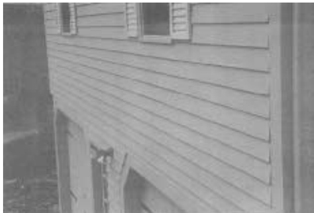
Figure 10. Hardboard vertical edges will swell and delaminate if not protected by wide enough cornerboards.
