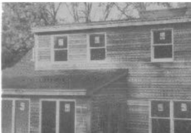
Figure 6. Gutters above might have prevented splashback from staining the siding where the lower shed roof connects.
