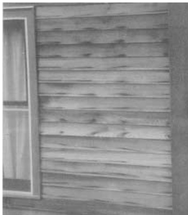
Figure 5. Uncoated or poorly coated nails look lousy when they bleed. The iron oxide also deteriorates the wood around the nail.
