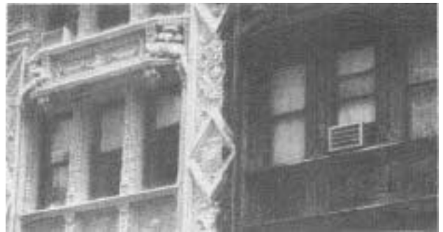
Two-stage chemical cleaning (alkaline) prewash and acidic cleaner from ProSoCo, reveals the rich terra-cotta facade under years of New York City grime on the Alwyn Court House. Chemical cleaning can be economical and safe to the building. It's applied with a roller, brush, or low-pressure spray.
