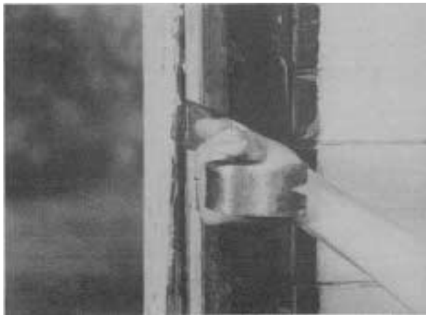
With a flat bar, pry off the parting bead to free the top sash.
