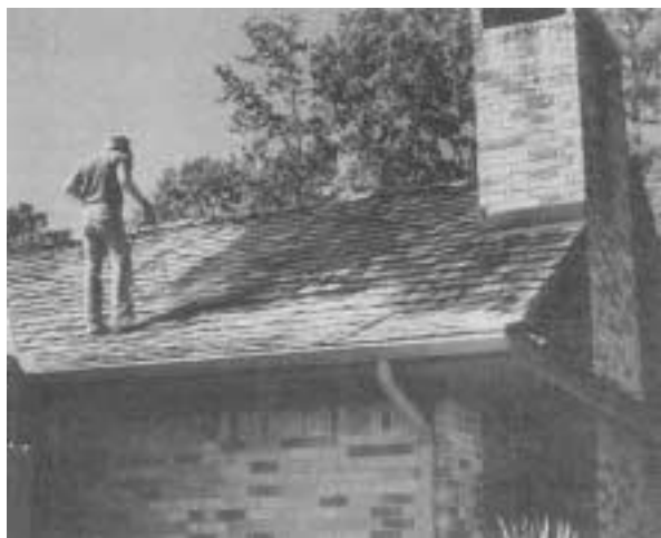
After power washing and repairing this red-cedar roof, a worker sprays on Cunapso 5, which will keep it free of mold, lichen, and decay for up to five years.
