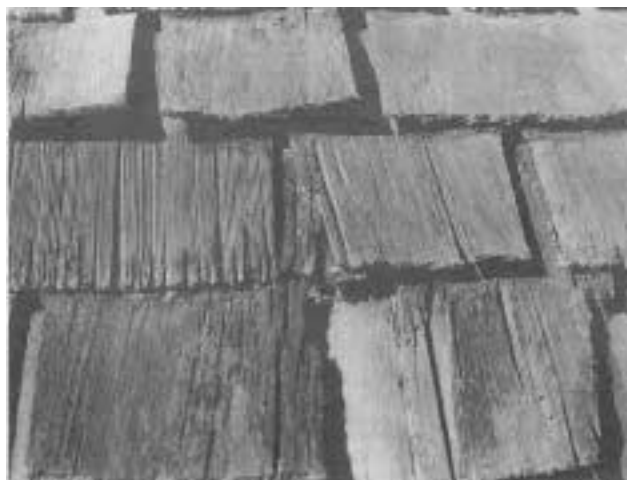
These 12-year-old shingles from an arid climate suffer more from sunlight than wood decay: the UV breaks down the wood, leading to cupping, curling, and splitting. Oil-borne treatments are needed to fight these drying stresses.
