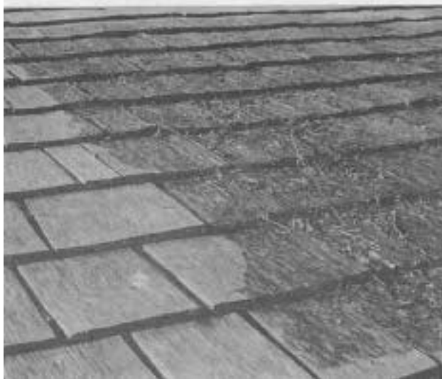
Power washing with water (top), popular in California, restores cedar roofs to their original brown color (bottom), even if they are covered with bleach-resistant lichen and algae. Power washers can be rented at many paint stores. Roofs that are merely discolored can be bleached, instead, which is easier on the wood.
