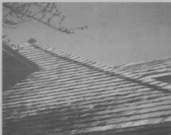
Pressure-treated pine shakes will weather to an attractive buckskin tan — the same color as pressure-treated wood—regardless of climate.
