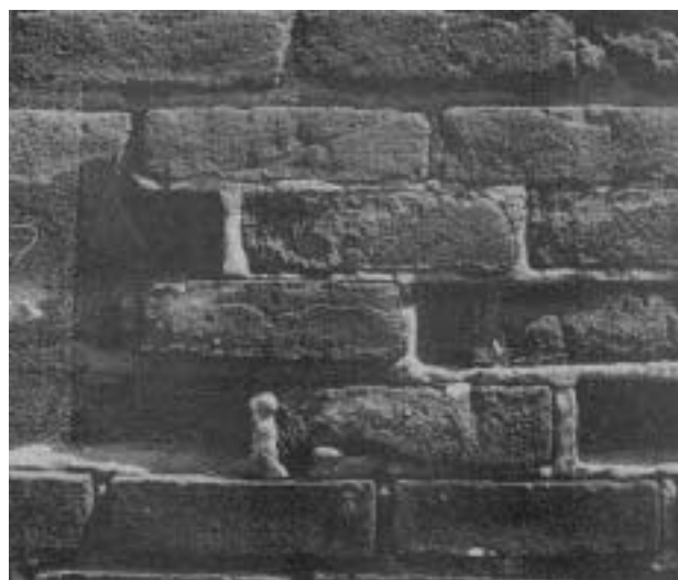
This brick suffered the double whammy of sandblasting, and repointing with hard portland-cement mortar. The results (left): deteriorating brick and protruding mortar joints. The diagram (right) shows the effects of temperature change on lime mortar and cement mortar in old masonry.
