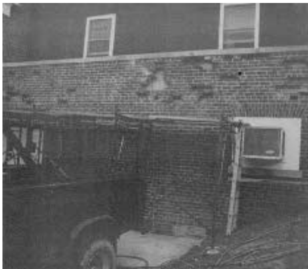
To repair this brick-veneer facade, author Michael Watson had to remove and replace a number of damaged bricks before repointing.
