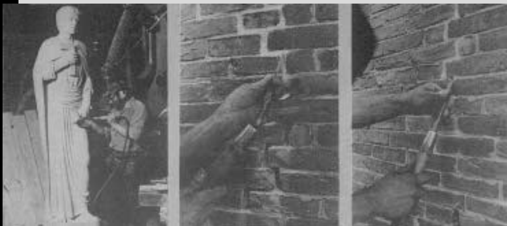
The Trow & Holden pneumatic chisel was developed for sculpture (left), but can also remove old mortar quickly and with little fatigue to the worker. The worker maintains precise control by manipulating the loose-fitting chisel (center), and controlling the pneumatic back-pressure with his other hand. Vertical joints are easily cleaned (right), without harming adjacent brick—a real problem with grinding equipment.
