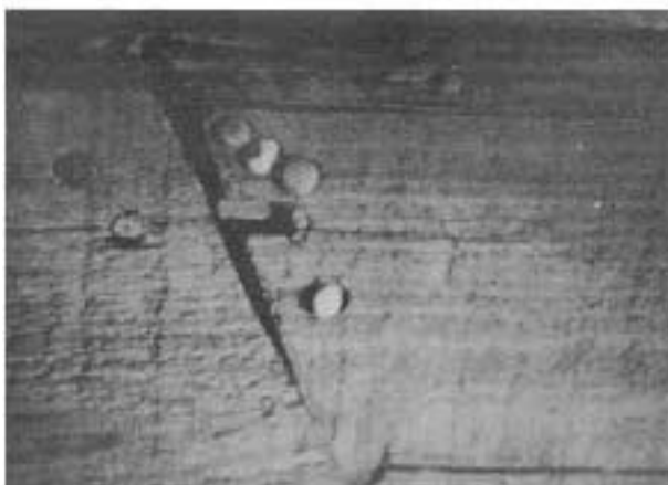
Some carpenters just can't bang in enough nails. Board-and-batten siding (top) is prone to splitting if boards up to 8 inches wide get more than one row of nails. The channel-rustic (center) isn't going anywhere, but should have been nailed only at the studs. Do you think they put enough nails in the T&G butt joint (bottom) to keep it in place?
