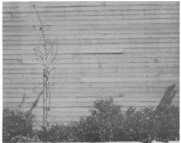
In general, staples will not provide the corrosion resistance or withdrawal strength needed for wood sidings (left). As for nails, (right) 1½ inches penetration into studs would have prevented these pullouts.
