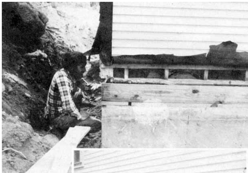
Repair worker Dana Myrick surveys moisture damage to the sill and band joist on a ten-year-old house in central Vermont. Standing water in the crawlspace, negative grading around the perimeter, and a bath fan exhausted into the attic all contributed to the problem.
