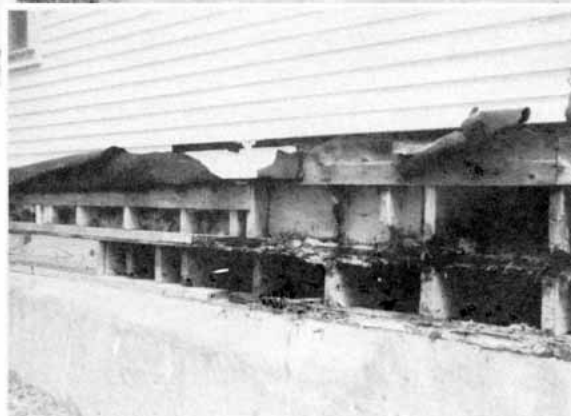
Repair worker Dana Myrick surveys moisture damage to the sill and band joist on a ten-year-old house in central Vermont. Standing water in the crawlspace, negative grading around the perimeter, and a bath fan exhausted into the attic all contributed to the problem.
