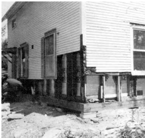
Figure 3. A simple half lap is the easiest joint to use where the new sill reaches the corner of the building. You need to cut a mortise if you want to preserve a tenon at the bottom of the corner post.
