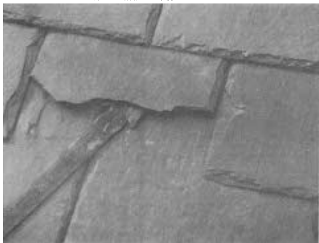
To remove the damaged slate, first hook the ripper (left) on one of the two nails holding the slate. Then hammer downward on the ripper (center) to cut or pull the nail. Next drive in a slate hook (right) to hold the replacement slate.
