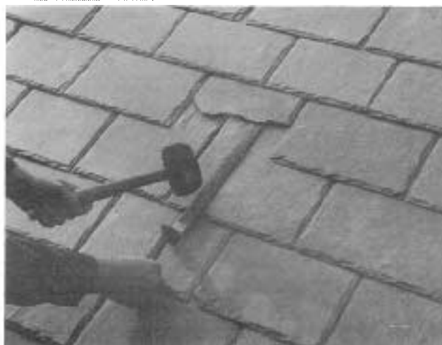
To remove the damaged slate, first hook the ripper (left) on one of the two nails holding the slate. Then hammer downward on the ripper (center) to cut or pull the nail. Next drive in a slate hook (right) to hold the replacement slate.
