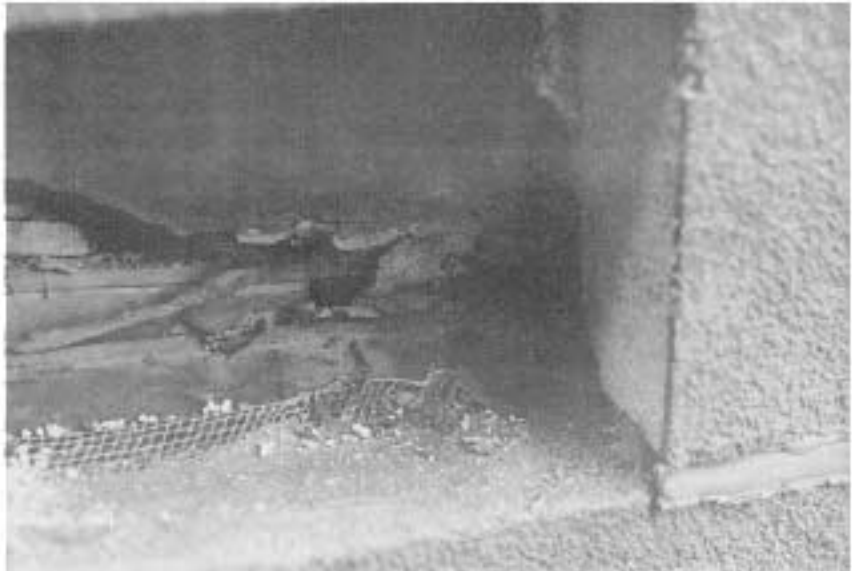
This structure looked good on the outside, but moisture readings (left) indicated wet sheathing. Further investigation revealed that some buildings had large areas of damaged and delaminated sheathing (right) from water that penetrated at trucks and horizontal sealant joints.
