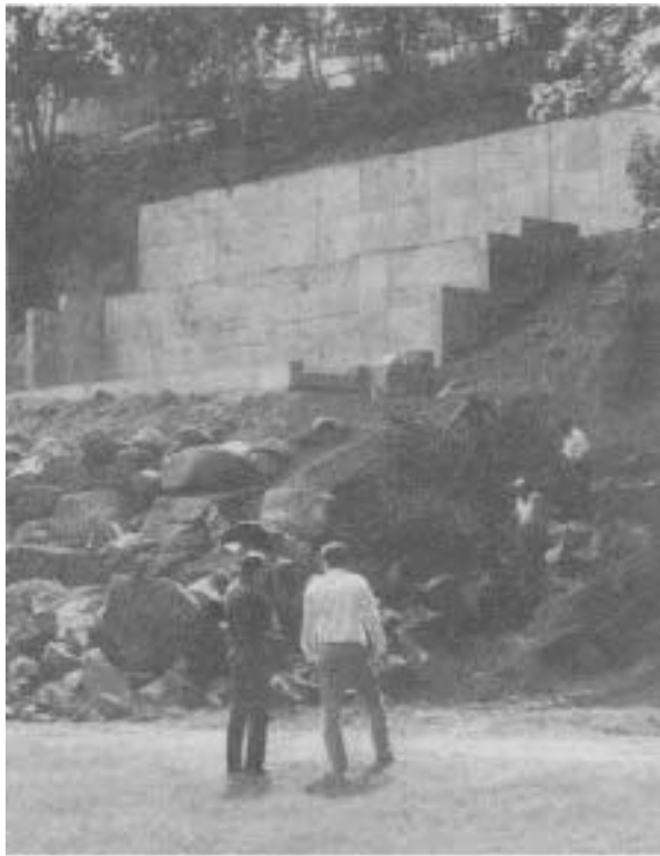
A two-tiered slab on stepped footings enabled the builder to fit two townhouses onto this steep and narrow urban site.
