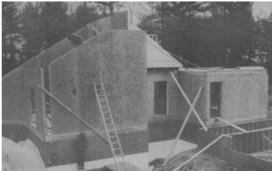
Builders assemble a custom saltbox using panels provided by Branch River Foam Plastics. Panels are cut in the field according to shop drawings that Branch River supplies for each home.
