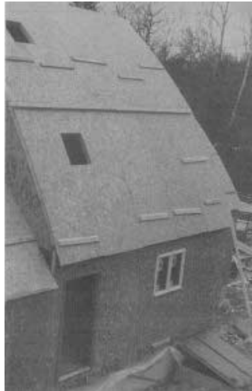
A fresh polyurethane panel rolls off the machinery at Winter Panel Corp., in Brattleboro, Vt. (left). The machinery foams the insulation in-place between two long waferboard faces. By curing the panels in a curved mold, Winter can create the bowed panels used in his bow-cape design (right).
