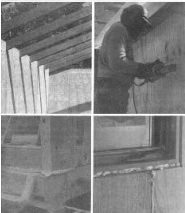
Any design, such as the classic colonial above, is possible for Cheney Building Systems, in New Berlin, Wis., which customizes panels for each home. Typical details include (clockwise from top right) chainsaw window cutouts; foamed-in-place windows; panels continuous to sill; and rafters sitting in notches. When trusses are used, they sit on a let-in 2x4 top plate.
