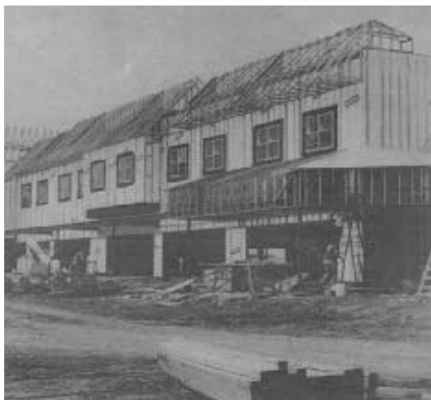
The Wallframe system from Arco Chemical is not a stress-skin, but uses an EPS core set in a galvanized steel frame. The system was chosen for the second floor of this shopping center in order to meet a tight production deadline.
