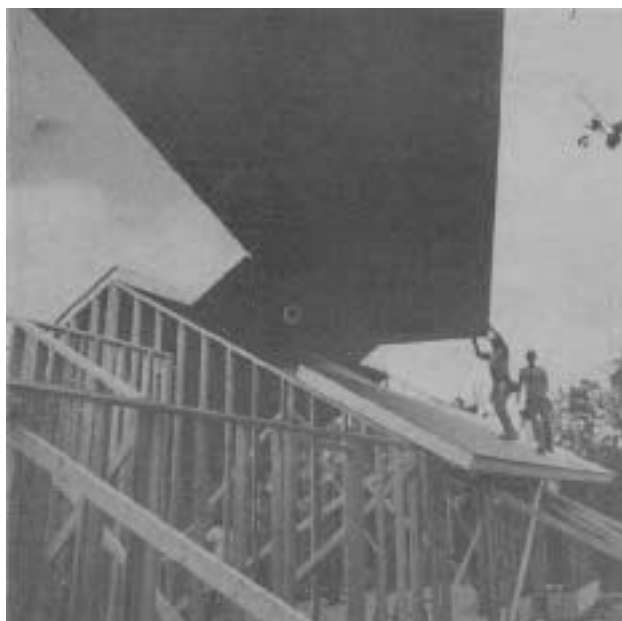
Oklahoma contractor Charles Harra stick-builds walls, but uses oversized 8x28-foot panels for the roof (left). Because the R-30 panels can span 14 feet, they yield open and flexible interior spaces, in addition to top energy performance. The eaves are trimmed out traditionally (right).
