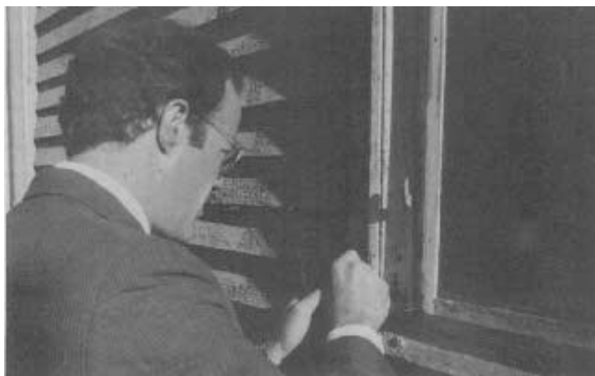
With a trained eye and lightscope, author Samuel Perry examines the siding of the historic Weatherbee farmhouse, in Westwood, Mass., to determine type, colors, and number of layers of exterior finish.
