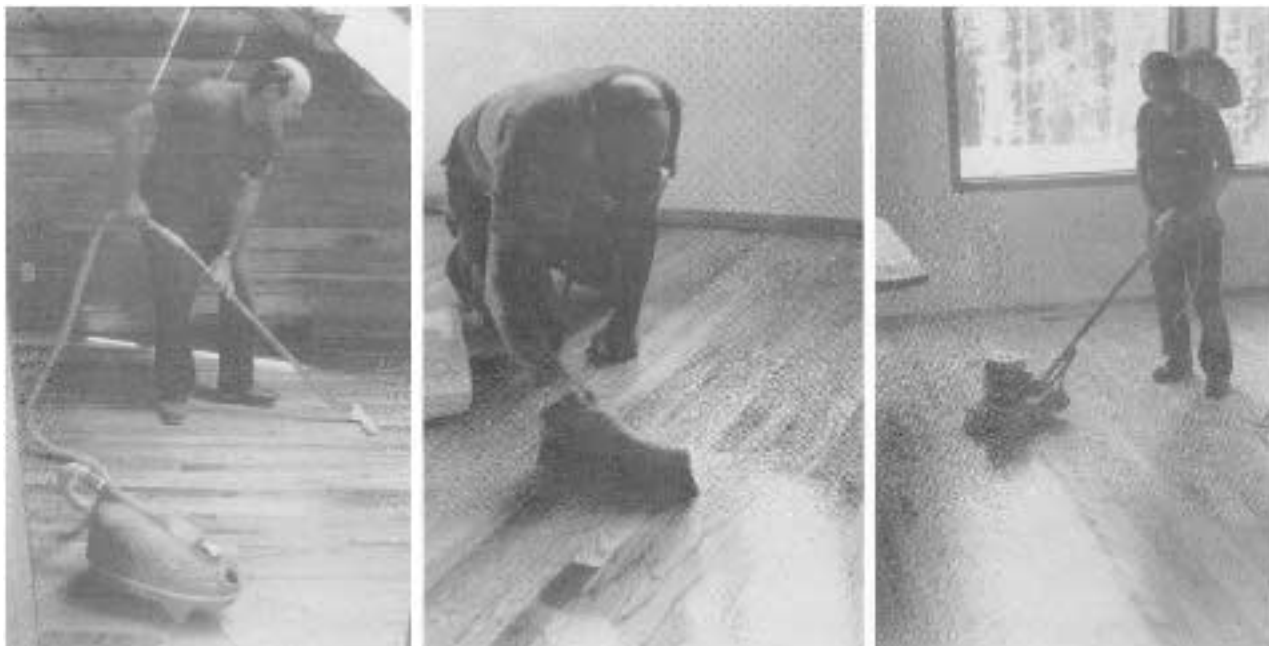
Swedish-type finish: Vacuuming removes all dust (left). Next, two coats of Glitsa's two-part sealer are applied (center) with a 12-inch china-bristle brush, as shown, or a lambswool applicator. A light screening (right) precedes the finish coat.
