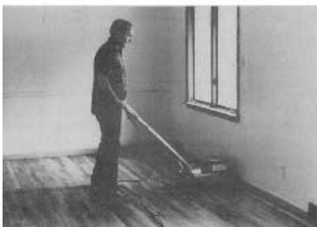
Using a special foam-backed mohair applicator, a floor finisher applies a coat of water-based urethane. The applicator is designed to apply a thin, uniform coat, which this type of finish requires. Between coats, the floor is lightly screened (bottom) to smooth the raised grain.
