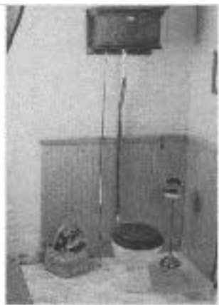
Older technology doesn't have to be inefficient: This pull-chain commode uses only 2½ gallons per flush.
