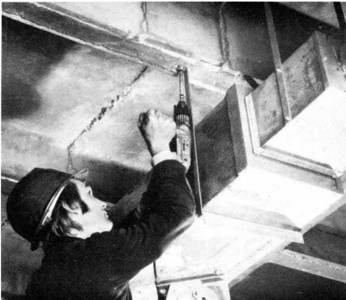
A worker fastens a duct hanger to concrete using concrete screws, which are inexpensive and fairly strong fasteners.
