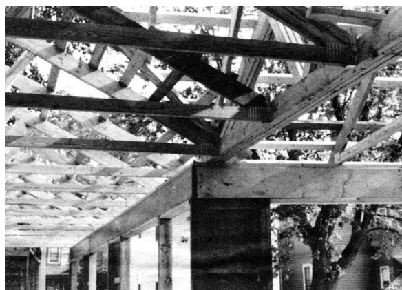
Figure 3. Three trusses are ganged to make a bearing beam at the inside corner of the building. Trusses with their tails cut off hang from the beam with joist hangers.
