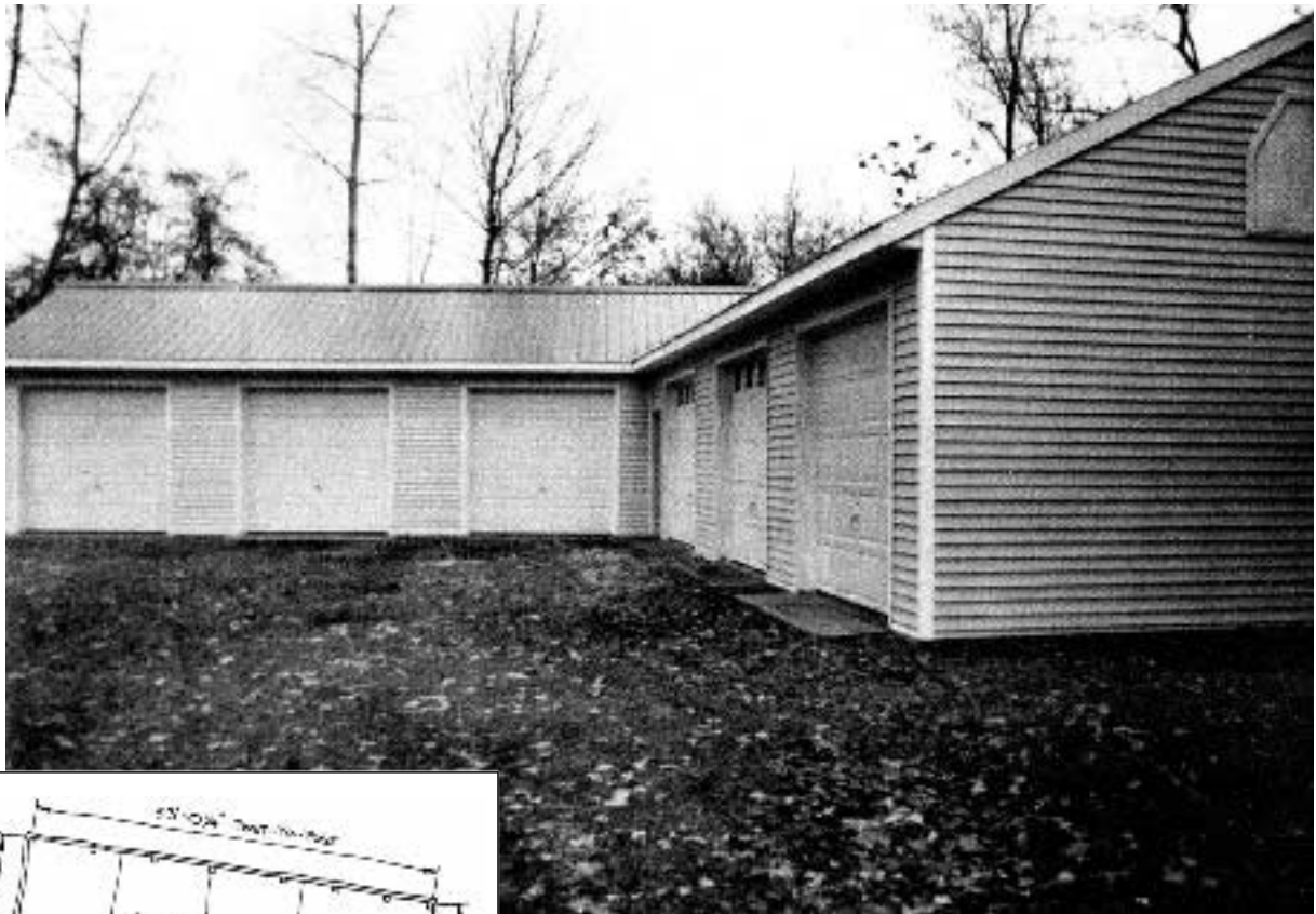
Posts on 8-foot centers allowed economical use of standard lumber sizes. Vinyl siding was used on front and gable ends for a traditional appearance.
