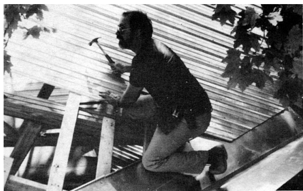
Figure 5. Metal roofing is installed with ring-shanked gasketed nails driven in the ridges, not the troughs. The valley was custom-fashioned from 26-gauge galvanized steel.
