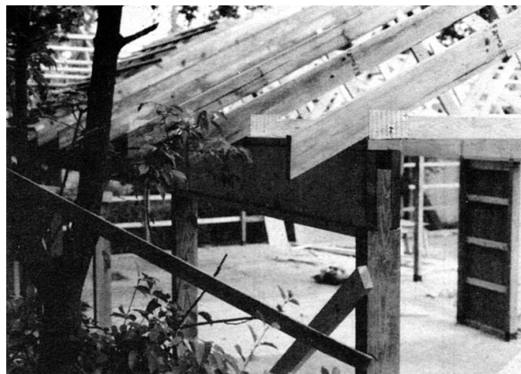
Figure 2. Double 2x12 headers are boxed in with 2x6s on the top and bottom. The 2x12s are notched onto the poles for a solid joint with no chance of splitting.
