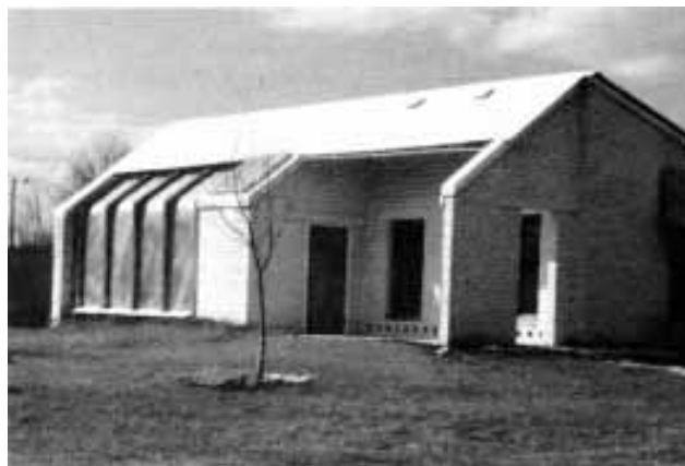
This community center in Carrizo Springs, Texas, uses bamboo trusses, and caliche-block bearing walls. The floors are mesquite wood, which is so populous in Texas, defolianters are sprayed to keep it down.
