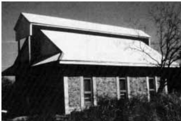
The straw walls in this Weberville, Texas, house are made by hand-tamping clay-coated straw into a plywood form. The practice is ancient, but the walls meet modern codes.
