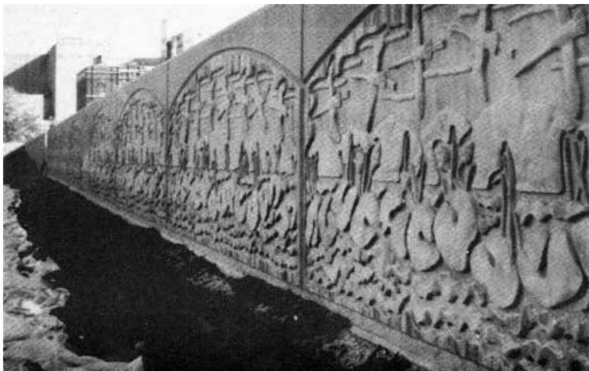
Form liners are available in 35 stock patterns, such as the one shown. Some liners have limited reusability, others can be used as many as 100 times.
