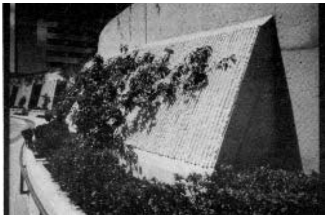
Form liners are available in 35 stock patterns, such as the one shown. Some liners have limited reusability, others can be used as many as 100 times.
