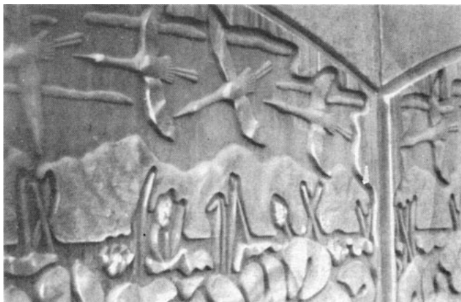
With some types of concrete-form liners, you can custom design your own pattern. This Winona, Minnesota river-wall features a concrete-formed scene of geese flying over a lily pond.
