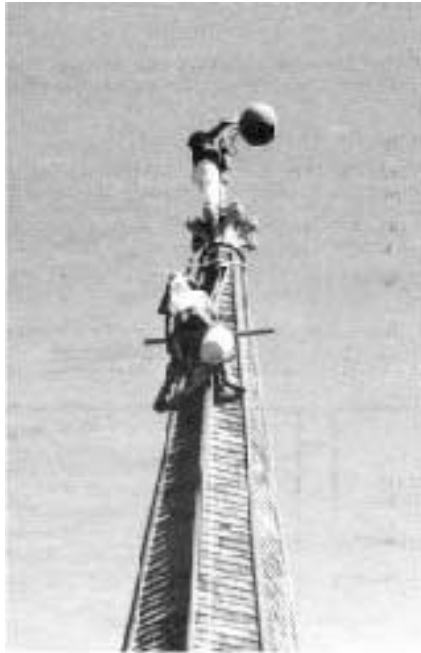
Michael Mastrototaro removes the ball from the weather vane spindle atop the Stratford, Conn., Episcopal Church. Greg Kilburn sits below him in a bosun's chair. Both steeplejacks are tied off with safety lines.
