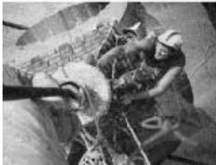
Using a block-and-tackle rope system, steeplejack Greg Kilburn hoists himself to repair molding on the Westminster, Vt., town hall.
