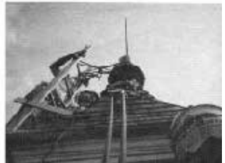
Using a stand-off ladder system, and wearing a safety belt, Mastrototaro inspects the slate on the Westminster town-hall steeple.
