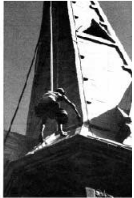
A bosun's chair, which hooks into the block-and-tackle, supports Paul Cloutier as he paints the metal roof on the Methodist Church in Burlington, Vt.
