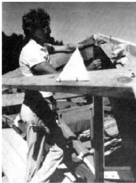
Figure 1. "Measure twice; cut once" takes on a new meaning with heavy timbers. But even with strings and 3-D joint models as guides, many timber joints needed fine tuning with chisels.
