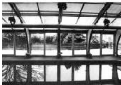
Figure 3. On an earlier project, we used sliding doors with fiberglass frames. Even with snow on the ground, they don't fog. The large roof windows operate by remote control.
