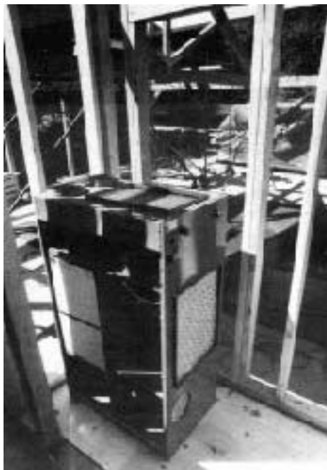
Figure 4. About the size of a drinking fountain, EDI's Ventrare unit combines heat distribution with heat-recovery ventilation.
