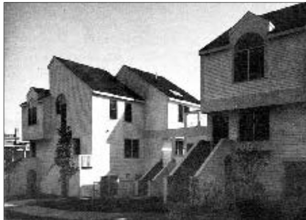
Figure 2. Cantilevers were used both to add interest to the building design and to increase living space. Also, because they act as a counterweight, they allow for longer interior spans.
