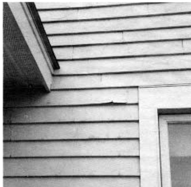
Figure 3. Where this roof and wall meet, the flashing leaked, and water saturated the clapboards, causing the paint to peel.
