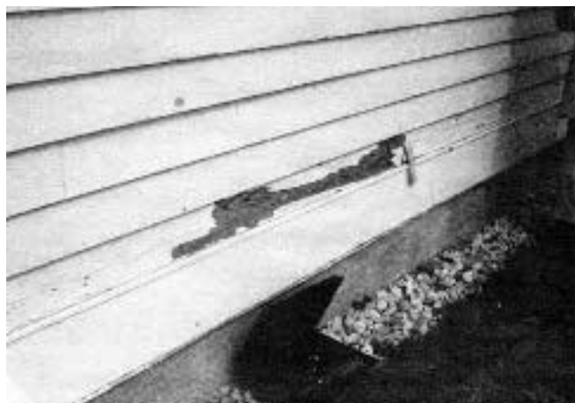
Figure 2. The flashing above the trim board was tilted inward causing the bottom clapboard to be constantly wet.
