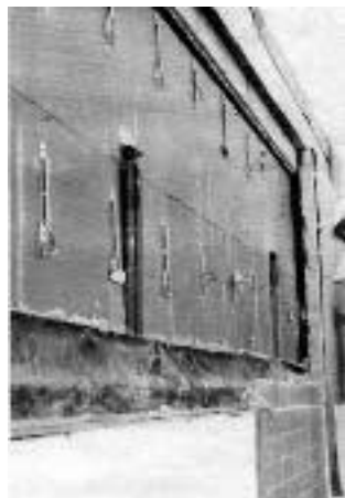
Figure 1. Elastomeric flashing was supposed to channel rain penetration out through weep holes in the brick veneer. But the flashing installation was sloppy and water was everywhere inside the wall cavity.
