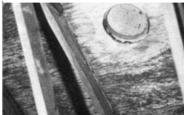
Basement moisture rose to the attic and condensed on the underside of the roof sheathing, causing black mold. The scuttle-type roof vent succeeded in protecting an area about one foot in diameter.
