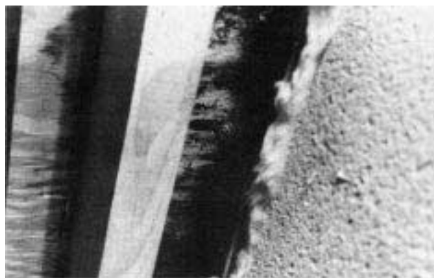
Condensed moisture rotted the floor sheathing in the band joist area of this Virginia crawl space. The rest of the floor sheathing, as well as the band joists, was unaffected.
