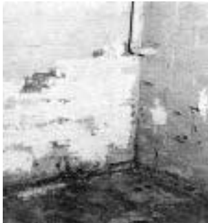
The basement wall coating, which was supposed to prevent seepage, was blistered and flaking off. The cause was less than obvious.
