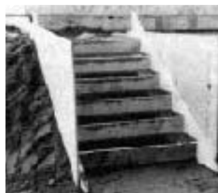
Figure 4. We used 3/4-inch plywood for the side forms, holding them in place with tamped sand. Sand also filled in below the stairs.
