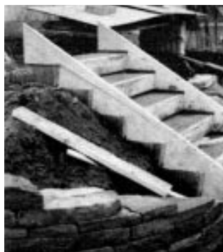
Figure 5. After finishing the treads, the plywood is pulled and the area is ready for landscaping.
