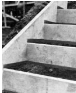
Figure 3. Riser forms are ripped with a 45-degree cut at the bottom to leave room to trowel the tread below.
