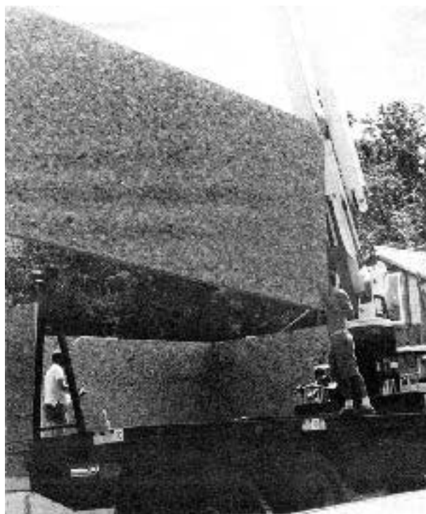
Figure 3. Structural foam panels can reduce labor costs without substantially increasing materials costs. It took one hour to close in the well-insulated exterior walls of this addition. Later, window-and-door openings were cut with a chain saw, and locally milled shiplap was applied as an economical siding.
