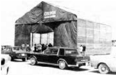
The steel-framed "Cocoon," which shields building sites from the elements, can withstand 60 mile per hour winds and heavy snow loads.
