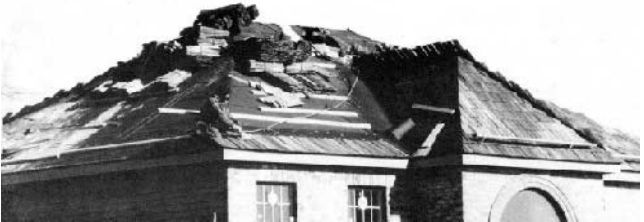
Complex roofs like this are the hardest to estimate. The trick is to divide them up into simple shapes
