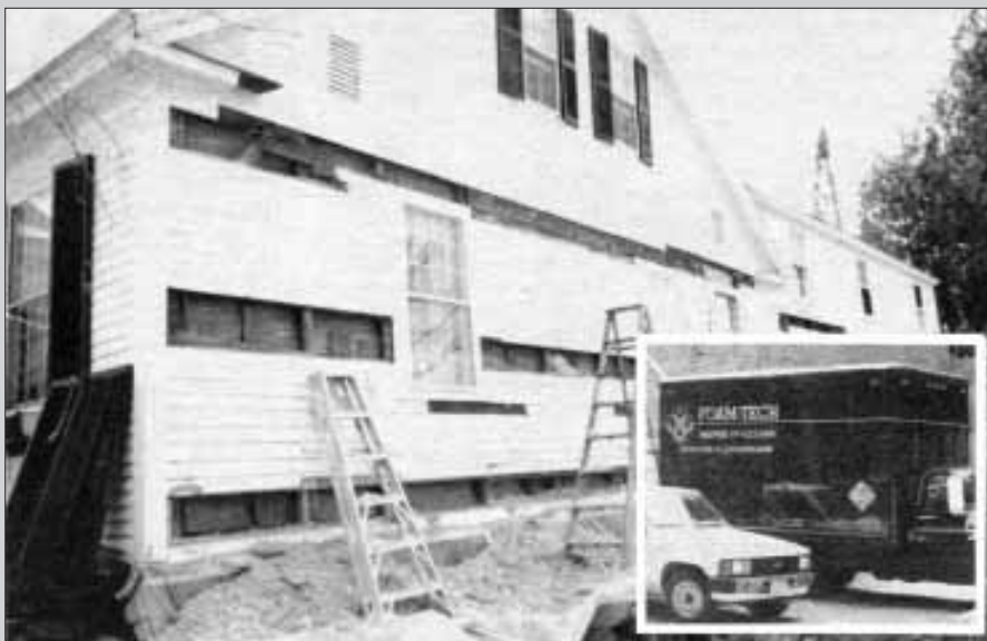
With walls opened and old insulation removed, this antique cape is ready for a dose of 20th-century foam — manufactured on board the truck (inset).
