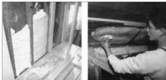
Figure 2. Because Air-Krete will slump, screen is used (left) to hold it in place in an open cavity. Similarly, screen with a temporary brace holds the foam between rafters (right). The installer is smoothing out the foam to keep it from bowing the screen.
