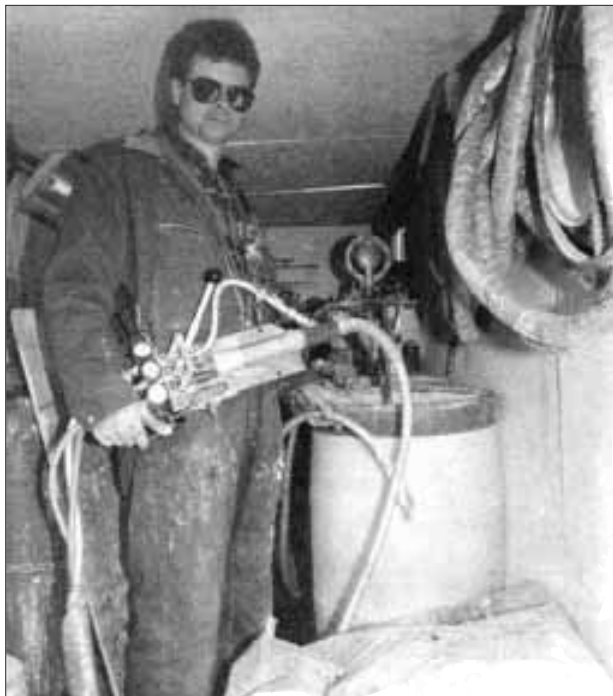
Figure 3. The Air-Krete gun precisely regulates the cement, foaming agent, and air to create the insulation.
