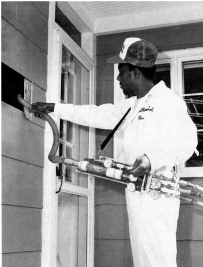
Dials and gauges regulate Tripolymer foam's chemical mix. The gun's precision and mechanic's experience make or break a foam installation.
