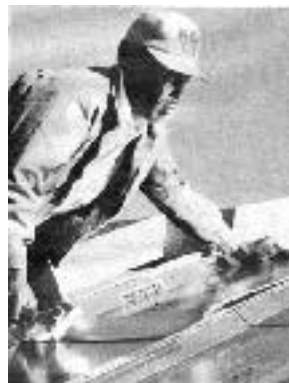
Parsec Retrofect Panels are pressure laminated panels covered with a radiant barrier material on both sides, and are designed to be used where hot and humid weather conditions exist over long periods of time.
