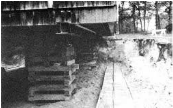
Figure 5. After jacking, the house was cribbed and continuous footing poured. The vertical #4 rebar will be wired to corresponding rebar in the block wall.
