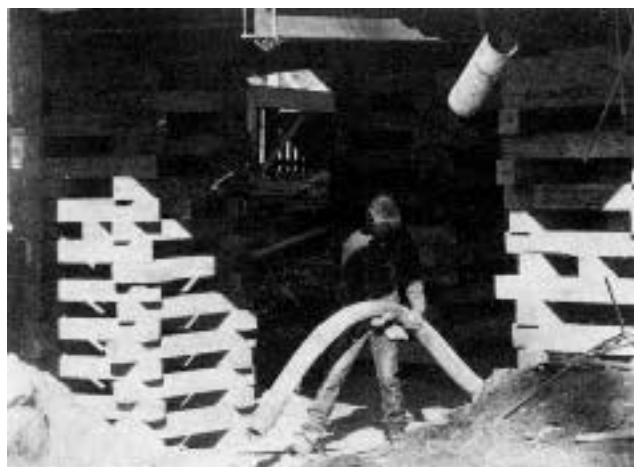
After this house was jacked up and supported with cribbing, a worker pumps in concrete for new footings. Repairing a failed foundation can cost a hundred times what it would have cost to do it right the first time.
