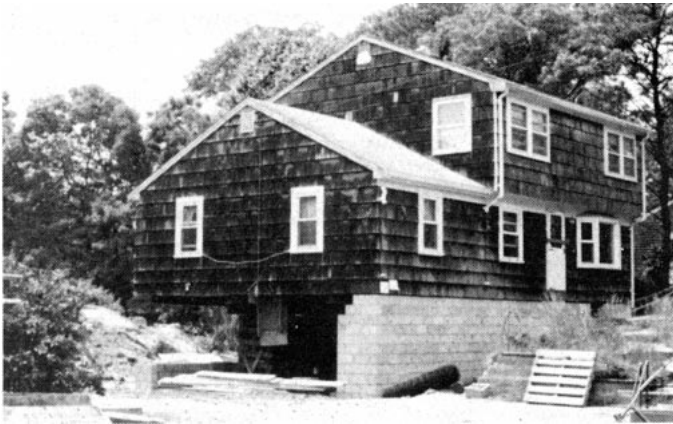
Figure 6. A concrete-cored reinforced block wall was built with Durawell-steel lattice every other course for lateral reinforcement. After the wall was in place, the house was lowered; cribbing and jacks were removed.
