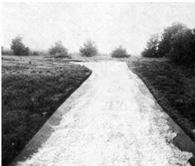
Figure 4. Geocomposites can drain under roads to prevent frost heave. This product, called Findrain (left), has special end caps that conduct the water into a 4-inch pipe, and then to a drainage ditch or storm drain. The road (right) with buried drains down each side of it, is ready for paving.
