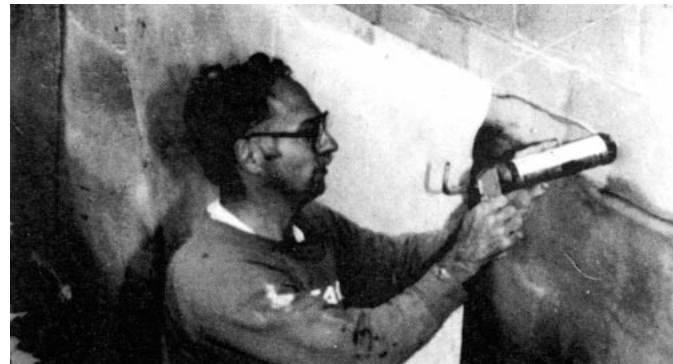
Figure 5. Expansive soils and hydrostatic pressure had caused the original block foundation to fail. The builders repaired the block wall, parged it with Thoroseal, and used a geocomposite to route water to an exterior sump. The result: no leaks in five years.
