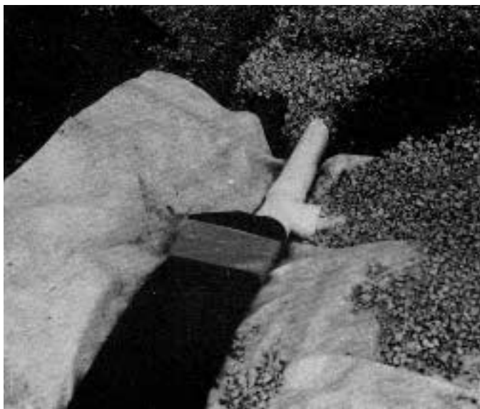
Figure 4. Geocomposites can drain under roads to prevent frost heave. This product, called Findrain (left), has special end caps that conduct the water into a 4-inch pipe, and then to a drainage ditch or storm drain. The road (right) with buried drains down each side of it, is ready for paving.
