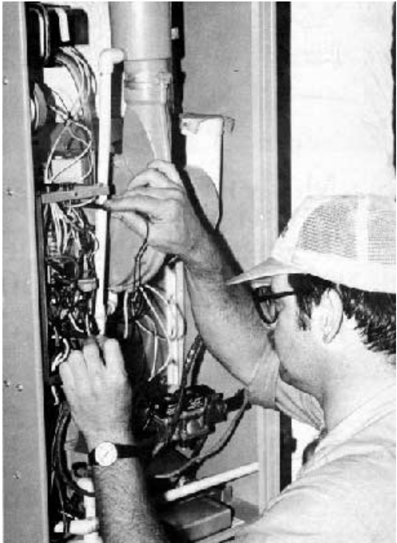
A furnace technician tests the controls on a condensing furnace during an annual tuneup. Special training and knowledge of electronics is needed.
