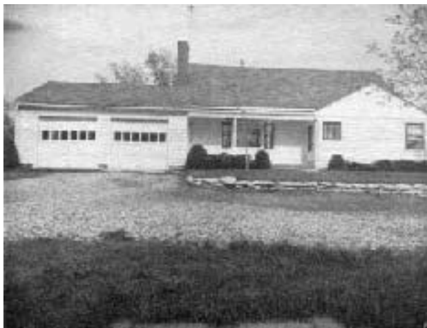
Figure 1. During construction, a lightning-protection system can be concealed from view and weather. The built-in system on this house shows only the 10-inch "air terminals" along the house's ridge.
