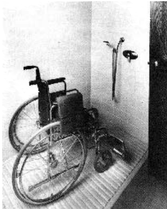
Figure E. This barrier-free roll-in shower with non-slip flooring and a low shower head and controls makes showering in a wheelchair much easier. Such a shower can often be fit in the space of a standard tub.
