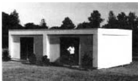
This prototype of the World House was erected last year, with volunteer labor, as part of a demonstration project for the United Nations. The materials cost $2,500, according to inventor Walter Feuchs.
