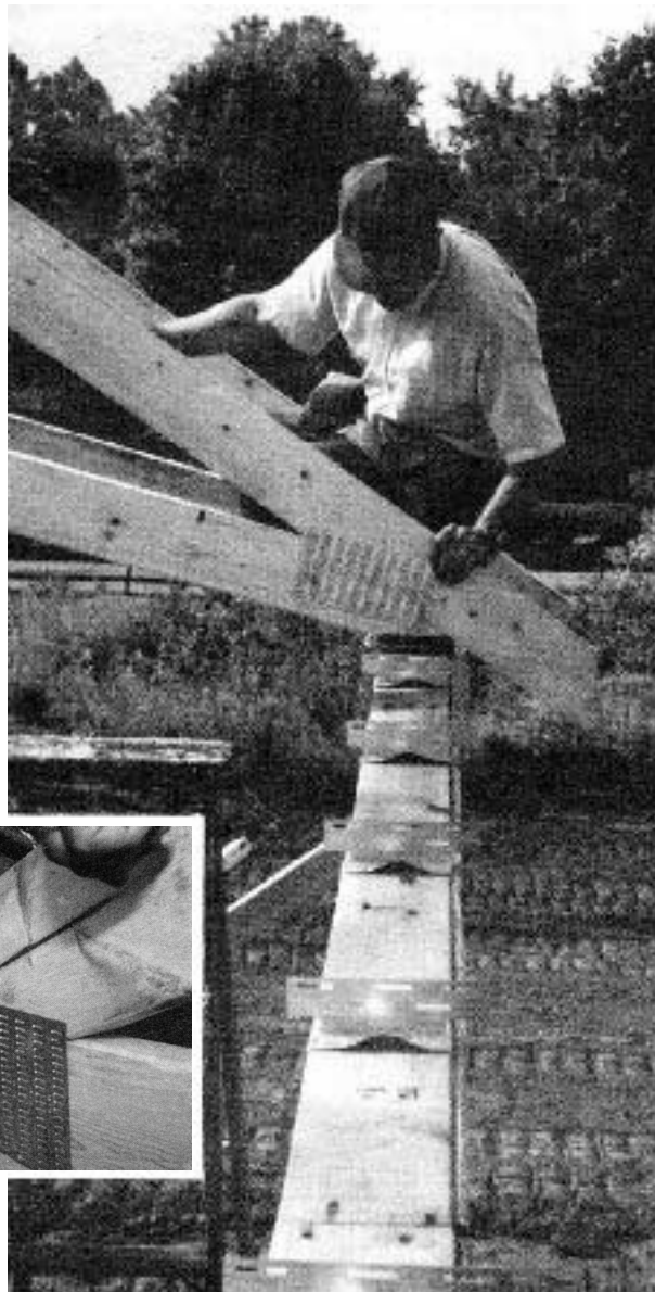
Up on the top plate, a worker sets a scissors truss into a specially designed anchor. The anchor (inset) prevents uplift while allowing the truss to slide back and forth as it deflects.
