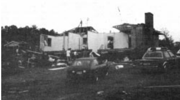
Insurance restoration jobs range from a porch that collapsed under a snow load (top), to a house damaged by a fallen tree (middle), and a home nearly leveled by a catastrophic storm.
