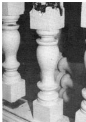
Figure 8. Balusters decay at block ends. Cut off these ends and repair with a doweled block to save the expense of turning new balusters.
