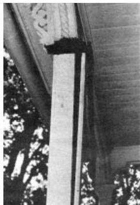
Figure 2. Columns wrapped in 1x stock conceal hidden damage. Take the columns apart very carefully because much of the material can be reused.
