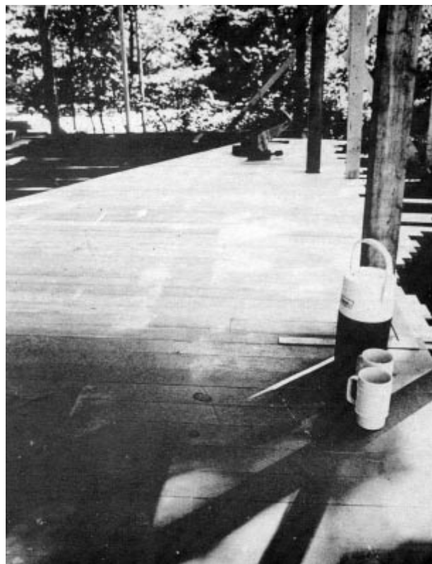
Figure 7. The thermos jug marks the spot where new tongue-and-groove porch flooring begins. Douglas fir flooring to match the old is still available.
