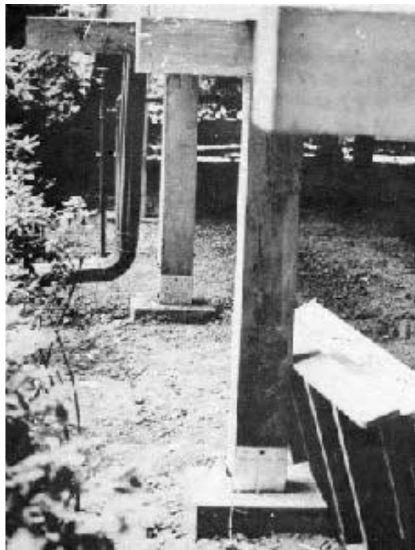
Figure 6. New posts are in place. The post-anchors will reduce future water damage.
