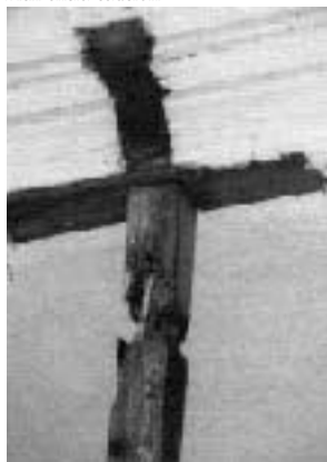
Figure 3. The post looks like it's been nibbled by beaver, but it's actually water damage.
