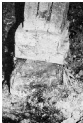
Figure 1. Dig down and you'll find surprises at footing level. This concrete footing, cracked apart, is resting on the original hunk of limestone.
