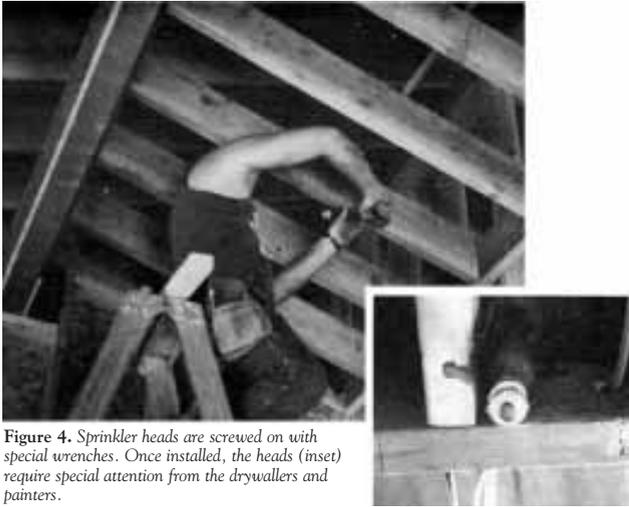
**Figure 4.** Sprinkler heads are screwed on with special wrenches. Once installed, the heads (inset) require special attention from the drywallers and painters.
