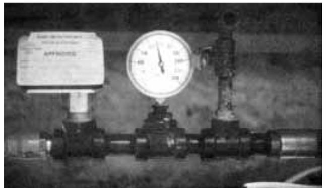
Figure 2. The riser, which feeds the system, also monitors and controls the flow of water. Large jobs may require several risers, each feeding an independent sprinkler array.
