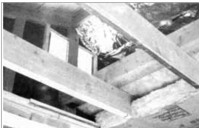
Figure 1. The three essential elements of a radiant barrier system are shown: adequate insulation, good ventilation, and a foil barrier. Not shown, but also important for cooling, is a light-colored roofing shingle.
