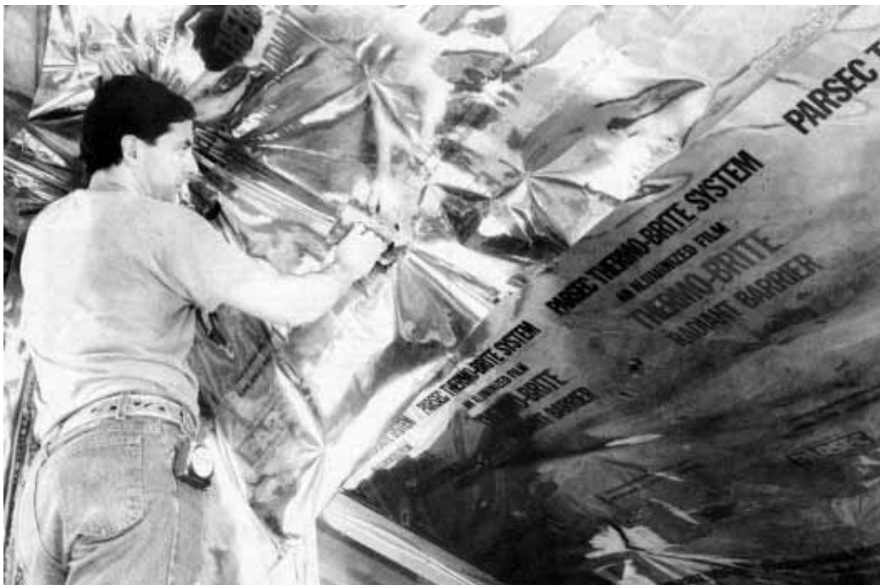
A worker retrofits a radiant barrier to the underside of rafters. The foil faces down to avoid dust accumulation.
