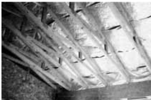
Figure 3. Draping the barrier over roof trusses before installing the roof sheathing is the favored approach of the Florida Solar Energy Center. Potential problems are scheduling hassles and wind during installation.
