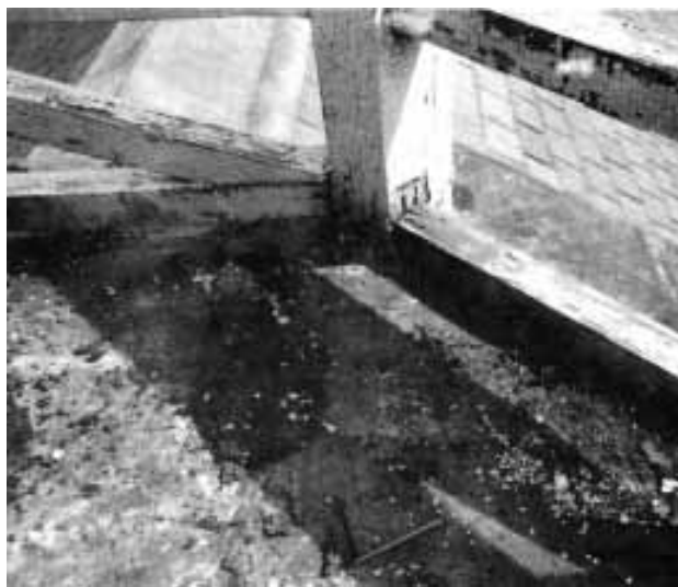
Figure 2. This railing, which fell to the deck and decayed, was beyond repair. The replacement used corrosion-resistant screws and nails, and the joints were sealed with Sikaflex caulk to keep moisture out.
