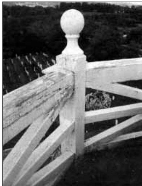
Figure 1. Because of the quality of the wood—old-growth northern white pine—this deteriorated railing was repaired rather than replaced. A pressure-treated replacement would likely have checked and warped.
