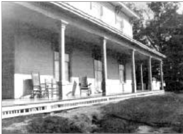
Figure 1. When built-in gutters were roofed over years ago, water flowed from the roof's edge, eroding the terrace.
