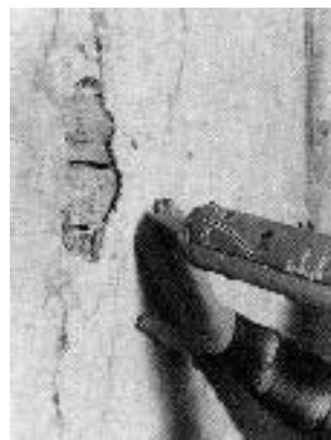
Figure 3. To reattach loose plaster to the lath, you can use a caulk gun to push specially formulated adhesives through pre-drilled holes.
