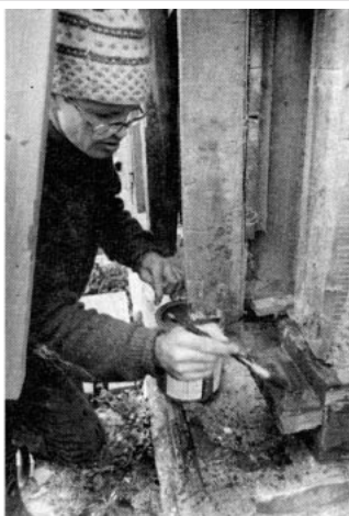
Figure 2. After treating the surrounding wood with Cuprinol fungicide (top) contractor Bill Noon, of Sanford, Maine, patches in a section of replacement sill built-up from 2x10 pressure-treated lumber. Notice how the first layer of replacement stock (center), and successive layers (bottom), are stepped back for a sturdy connection to the existing sill.
