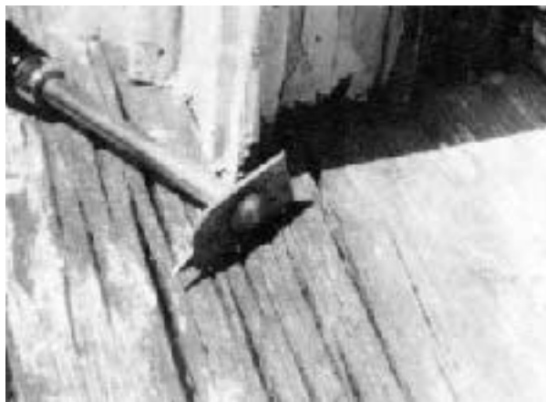
Figure 2. A special scraper helps clean out the checks in a weathered sill, before epoxy treatment.
