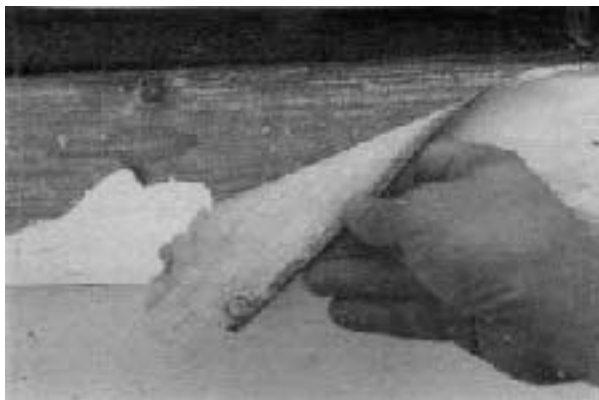
Figure 4. Peeling paint on the siding beneath the sill indicates high moisture content—and possibly a decayed sill.
