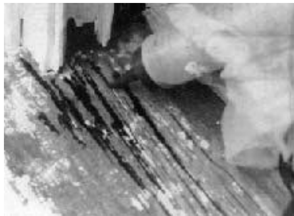
Figure 3. Epoxy consolidant is applied to the checks as a primer before they are filled with epoxy filler.
