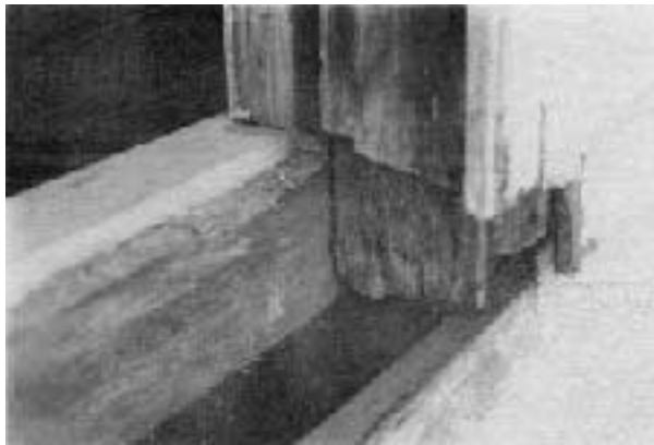
Figure 5. The decayed sill has been removed to determine the extent of damage to sill and frame. Note the rabbit joint at bottom of the frame stile.
