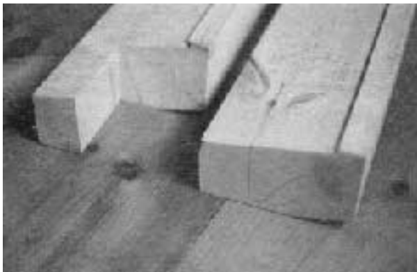
Figure 6. A new wood sill of eastern white pine is about to be screwed in place to repaired frame stile.
