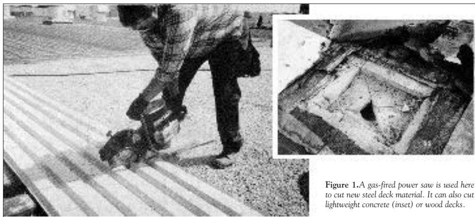
Thermosetting insulating fill. Make sure you don't change the roof slope when you cut through this deck. Patch in with tapered insulation.
