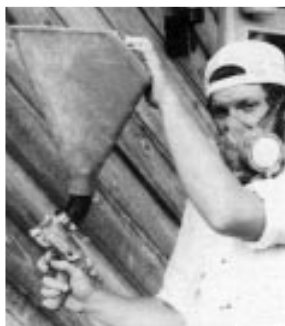
Figure 2. The spray gun's hopper is attached to the top of the gun and held on with a clamp. These guns are driven by a medium-duty 6.4 cfm portable air compressor. You can rent the whole setup (compressor and gun) for about $35 a day.
