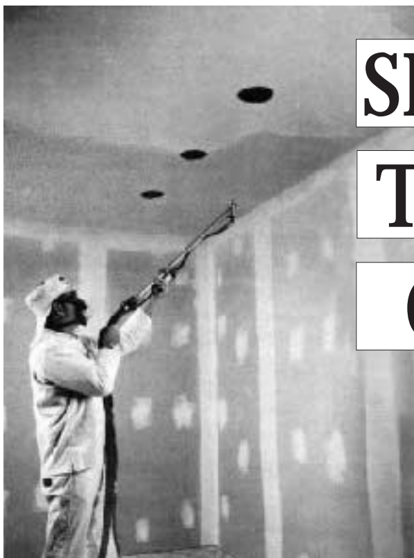
Sprayed-on ceilings can save you time on labor-intensive prep, and they can hide a lot of sins.
