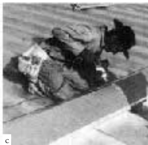
On a low-slope commercial roof: A worker screws metal purlins (a) through the old built-up roof. Panels are attached to the purlins with special clips (b) that allow for thermal movement. Movement is also accommodated at the ridge (c) by a flexible cap. To finish up, trim is installed at the rake (d) to be followed by the eave. (Manufacturer: Armco Building Source)
