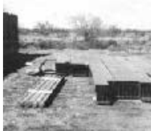
Figure 5. Open-profile panels nest for easy transport.
