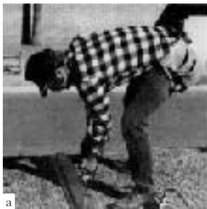
On a low-slope commercial roof: A worker screws metal purlins (a) through the old built-up roof. Panels are attached to the purlins with special clips (b) that allow for thermal movement. Movement is also accommodated at the ridge (c) by a flexible cap. To finish up, trim is installed at the rake (d) to be followed by the eave. (Manufacturer: Armco Building Source)
