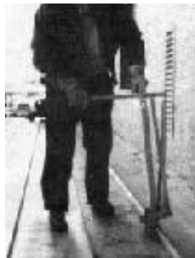
Figure 2. A crimping tool seals the ridges as tight as a tin can.
