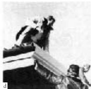
On a low-slope commercial roof: A worker screws metal purlins (a) through the old built-up roof. Panels are attached to the purlins with special clips (b) that allow for thermal movement. Movement is also accommodated at the ridge (c) by a flexible cap. To finish up, trim is installed at the rake (d) to be followed by the eave. (Manufacturer: Armco Building Source)
