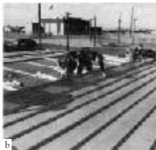
On a low-slope commercial roof: A worker screws metal purlins (a) through the old built-up roof. Panels are attached to the purlins with special clips (b) that allow for thermal movement. Movement is also accommodated at the ridge (c) by a flexible cap. To finish up, trim is installed at the rake (d) to be followed by the eave. (Manufacturer: Armco Building Source)
