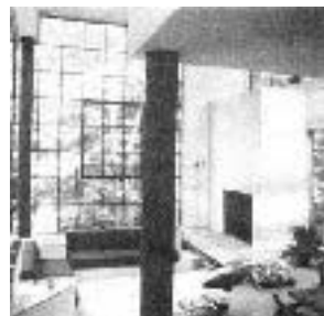
Floor-to-ceiling windows, which in this case use an industrial glazing system, dissolve the corner of the living room and visually extend the common area of the house into the forest. The dramatic quality of the room masks its relatively small size.
